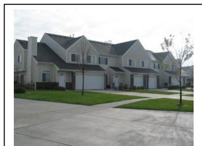
Example of Single-Family Attached
